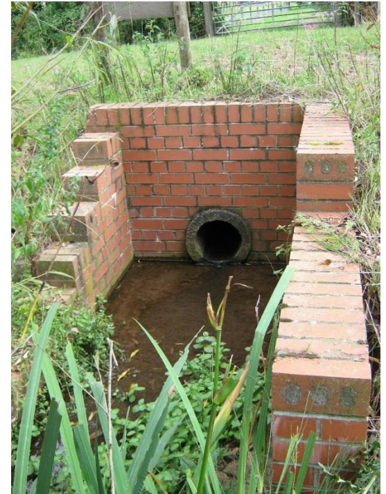
Culvert: Correctly sized, set at the correct level and with its' mouth kept clear
